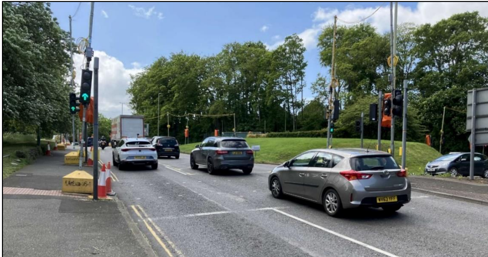
SRL Urban 64 temporary lights in operation at Harnham gyratory
