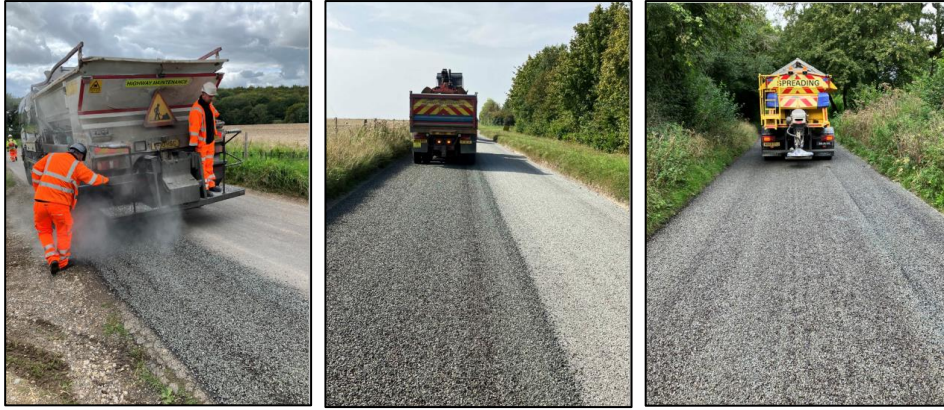
An extensive programme of surface dressing helps seal and protects the county's rural roads, and improves skid resistance.
